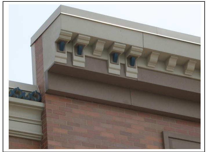
Top: This new cornice offers a simplified version of the original, which was destroyed by fire along with the historic building.
