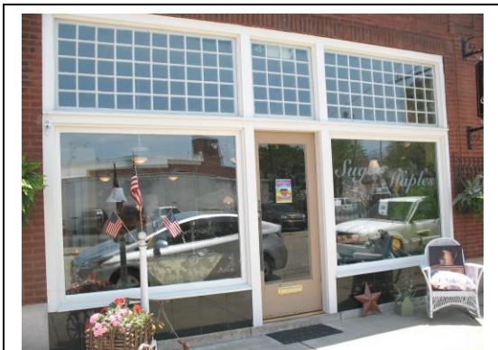
These multi-light transoms are important to this building's character, and should not be covered or removed.
