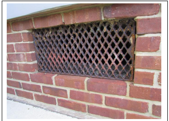
Top: The brick facing and salvaged iron grates help the foundation of the relocated Willey-Allbards House blend in with its new surroundings on West Chestnut Street.
