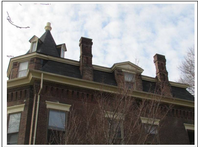
The chimneys – which feature inset panels and corbelling – and dormer windows, as well as the finial-topped corner tower, work together to provide great visual interest to the roofline of this West Riverside Drive home. .
