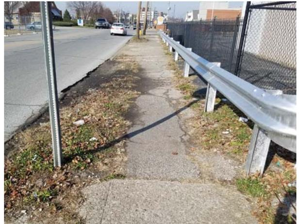
Deteriorating sidewalk and curb in the A&C segment
