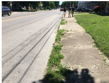
Cracked sidewalks
