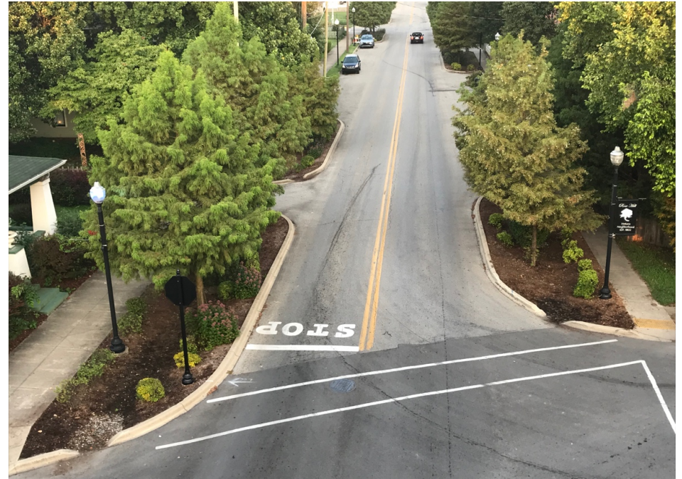
Curb extensions on Market Street help slow down traffic and collect stormwater.
