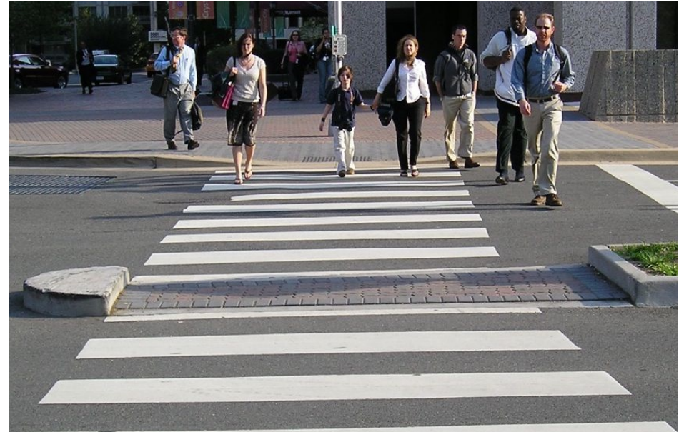
Continental striping at least ten feet wide is very visible to motorists. This crosswalk could have been bit wider.
