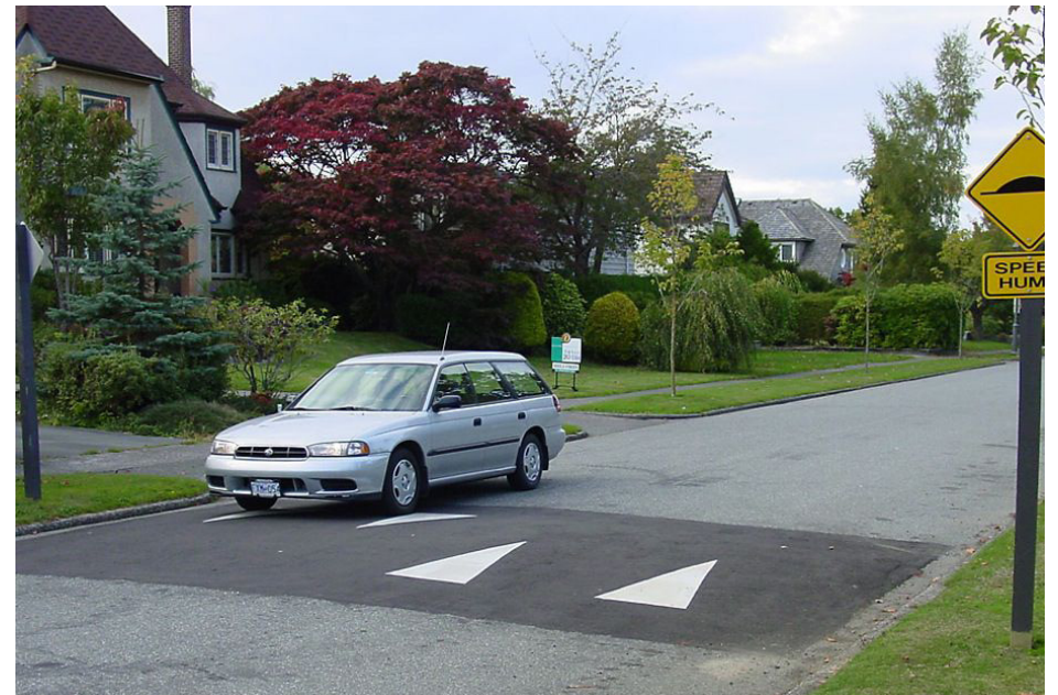
Speed humps are a reliable means of slowing down cars and are often used in combination with curb extensions and stop signs.
